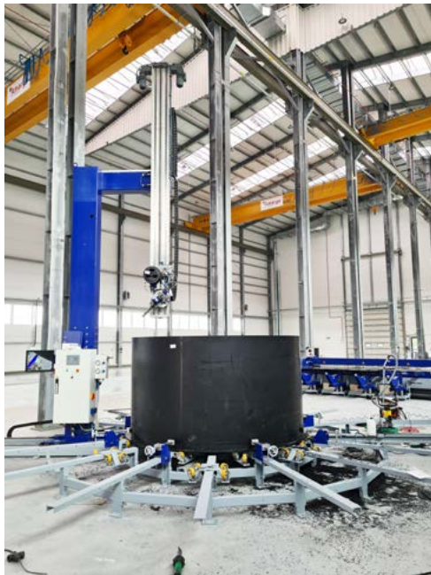
"Standard" technology using sheets of AmargTank ClassicWeld® plastic sheet
